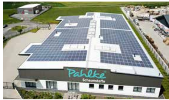
Our photovoltaic system, commissioned in May 2019.
