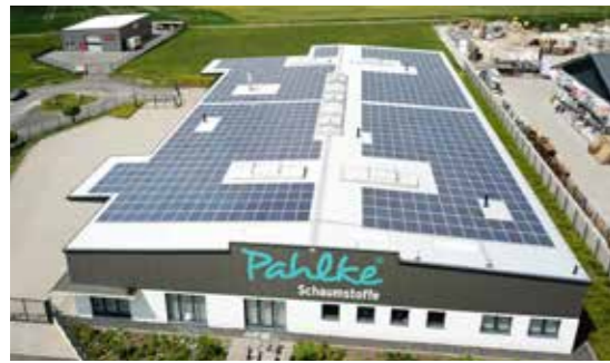
Our photovoltaic system, commissioned in May 2019.
